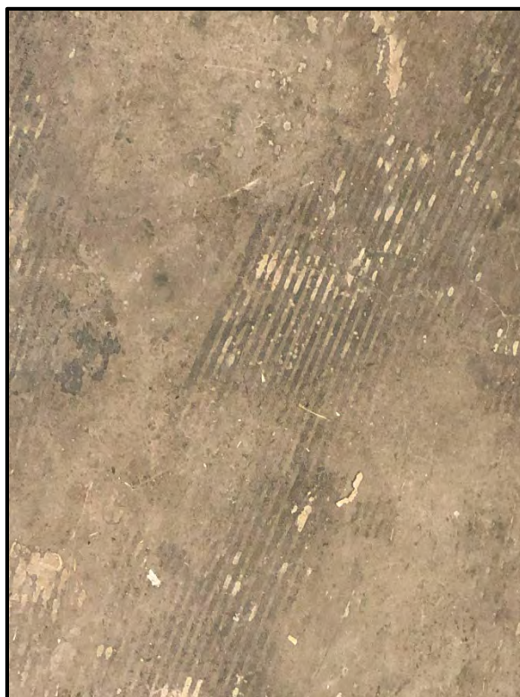
Asbestos Containing Black Floor Tile Mastic Remnants
