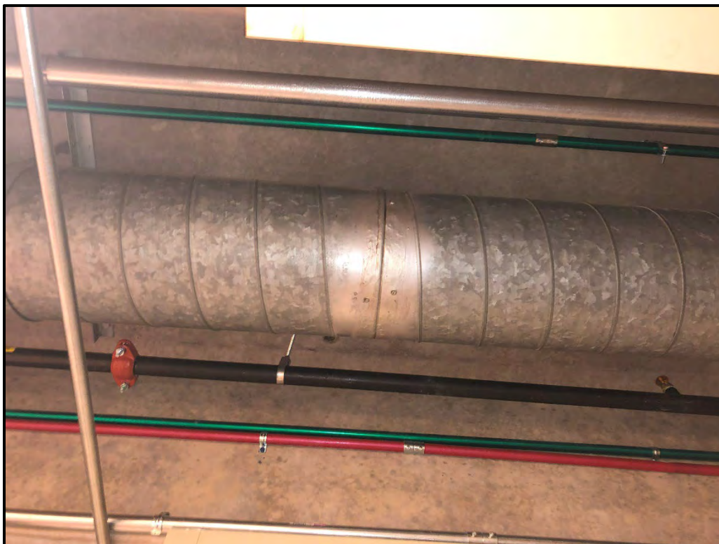
Asbestos Containing Duct Silver Sealant and Joint Sealant Caulk
